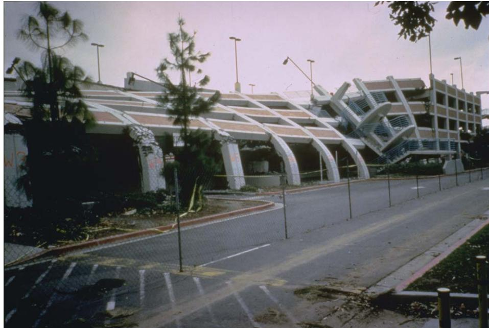
**Figure 2.6 Another view of the collapsed parking structure at the California State University in Northridge [20].**
