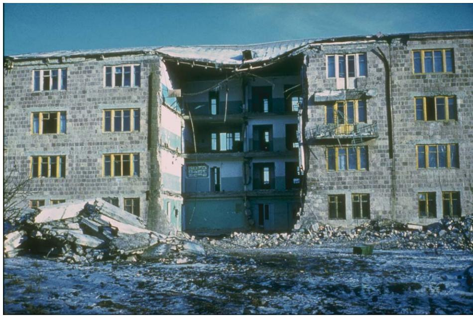
**Figure 2.3 Damage to a four-story building in Leninakan due to inadequate connection between precast floors and infill walls [20].**
