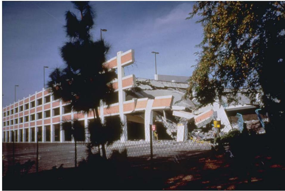
**Figure 2.5 Collapse of center columns, floors, and external moment frames of a parking structure at the California State University in Northridge [20].**
