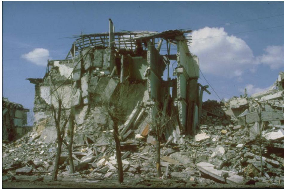
**Figure 2.2 Collapse of precast floor panels, leaving walls standing in a building in Leninakan [20].**
