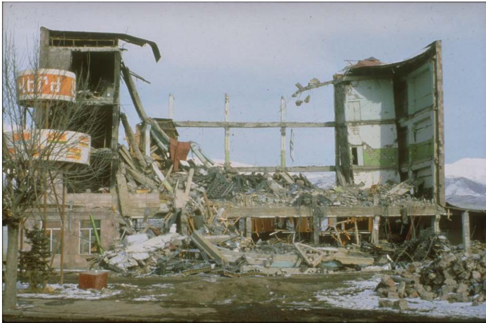
**Figure 2.4 Collapse of floor planks leaving external precast frames standing in a building in Spitak [20].**
