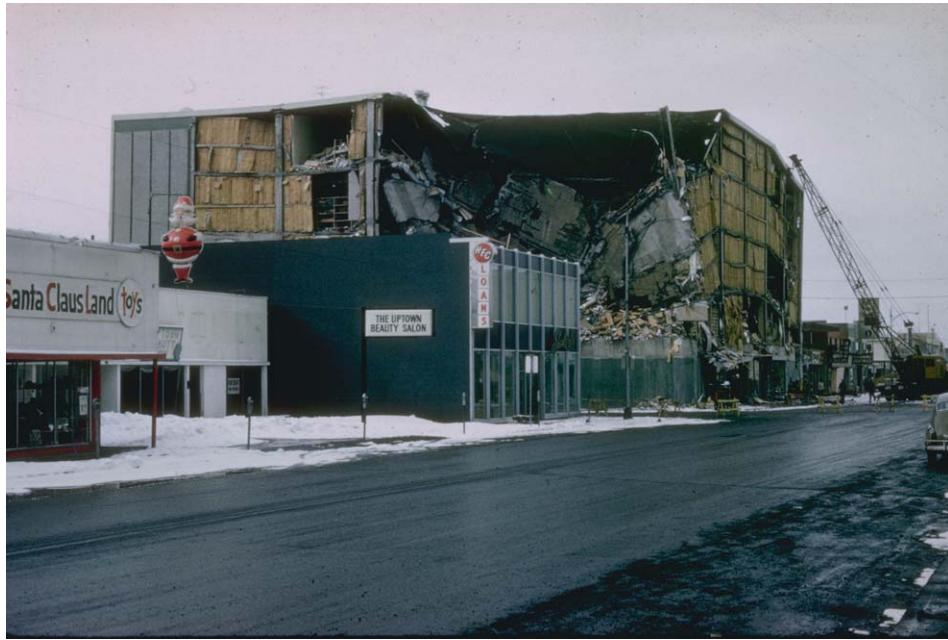
**Figure 2.1 Partially collapsed building that contained poorly connected precast floor panels [20].**
