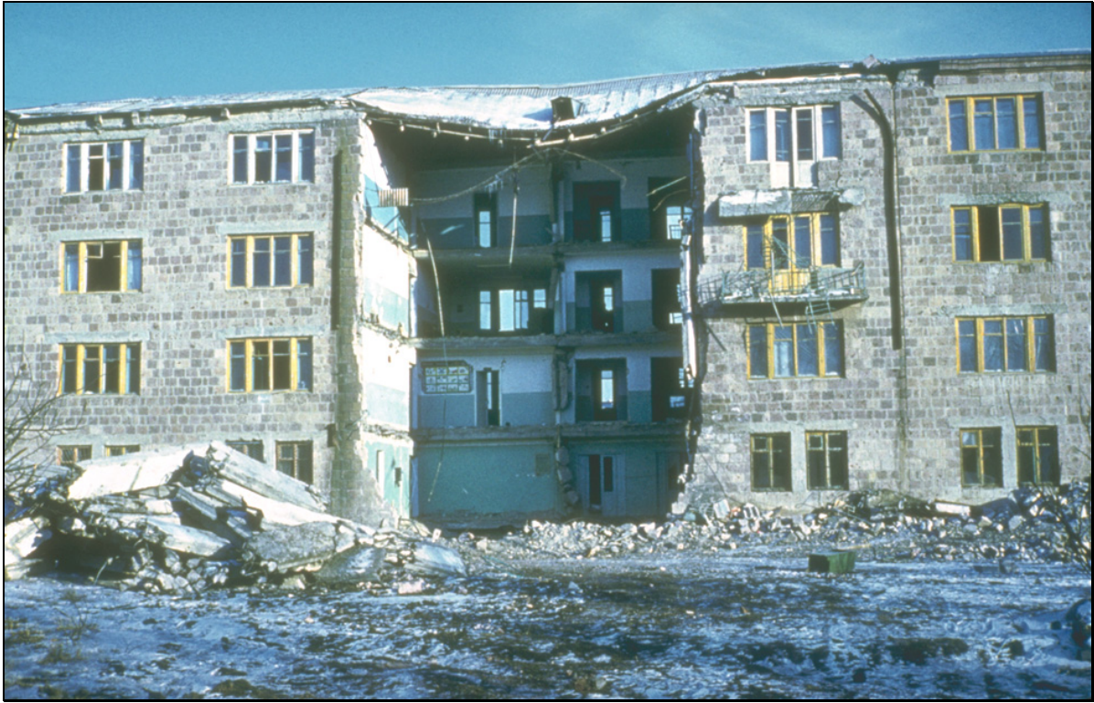
Figure 1.2 A partial collapse of structure due to inadequate connection details between precast floors and walls in the 1988 Armenian earthquake [1.3].
