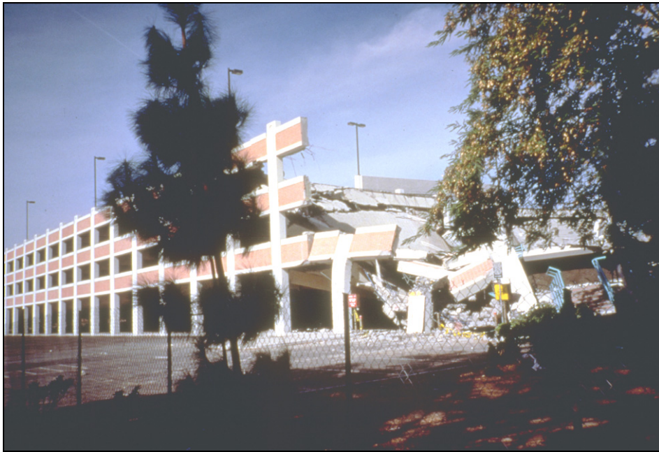
Figure 1.1 A view of a collapsed precast parking structure in the 1994 Northridge earthquake [1.3].
